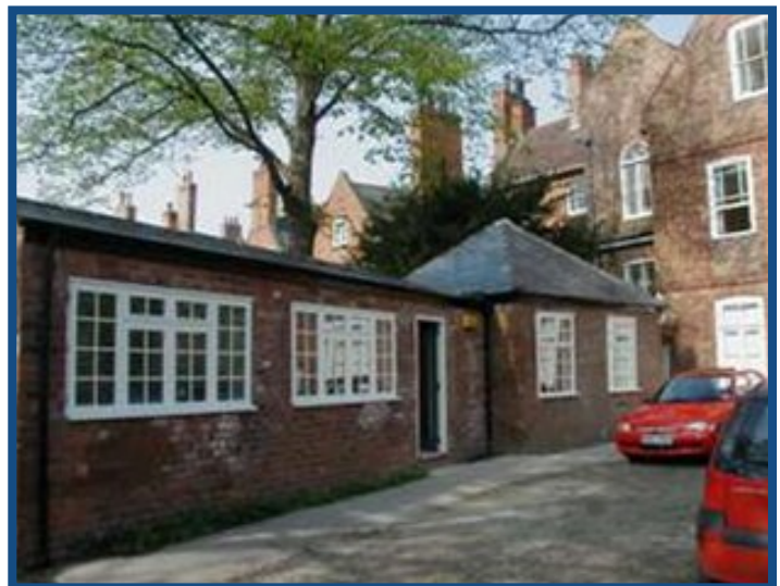
Rear self-contained Annex
