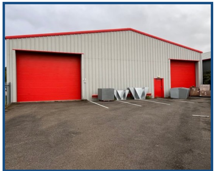
External View of Warehouse & Yard Area
