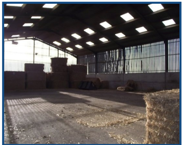
Internal View of the unit
