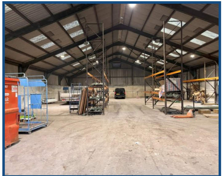
General Internal View of Unit
